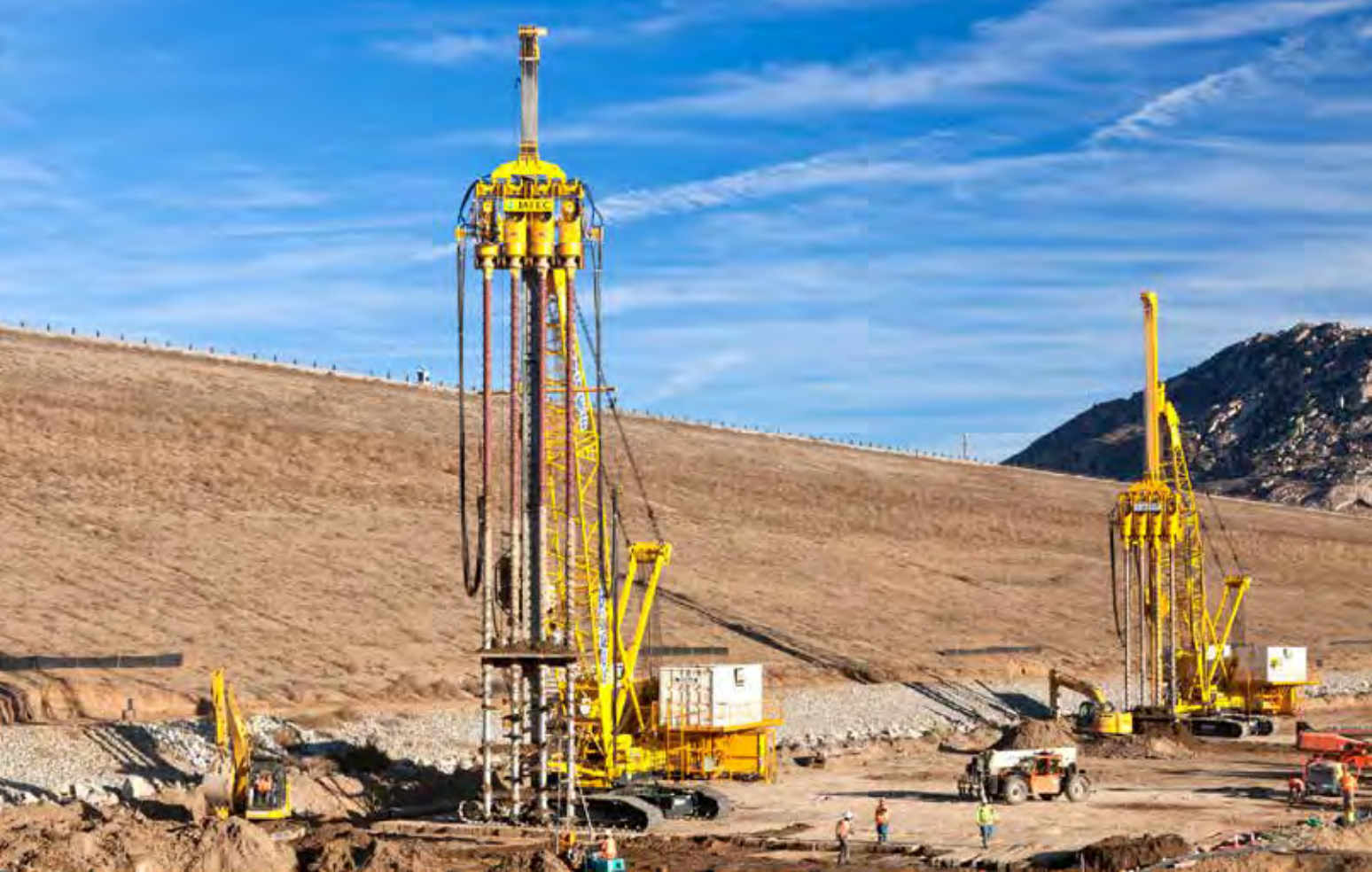
Figure 3. Deep mixing by the wet method using four-shaft, vertical-axis equipment at Perris Dam in California. (Photo courtesy of JAFEC USA Inc.)
