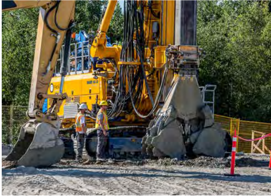
Figure 5. Deep mixing by the wet method using twin, horizontal-axis cutting and mixing wheels at BC Hydro substation in Burnaby, British Columbia. (Photo courtesy of Pacific Ground Engineering.)
