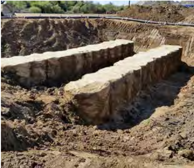
Figure 4. Excavation of test/demonstration section at Perris Dam. These elements were installed by the wet method using four-shaft, vertical-axis mixing equipment. (Photo courtesy of California Department of Water Resources.)
