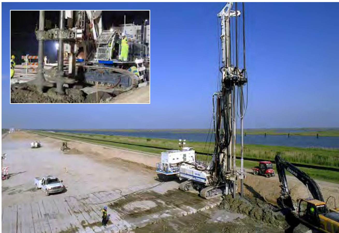
Figure 2. Deep mixing by the wet method using twin-shaft, vertical-axis equipment at earthen levee LPV 111 in New Orleans. Inset shows mixing blades in operation. (Photos courtesy of TREVIICOS.)
